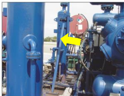
Figure L.19: Angle brace used to detune a scrubber natural frequency.
