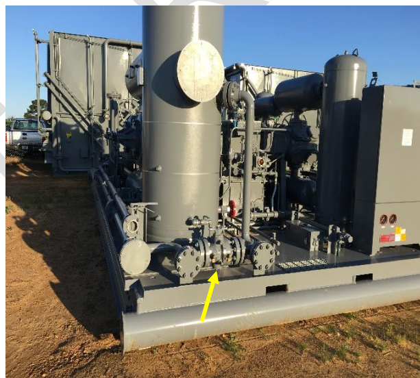
Figure P.8: On-skid startup bypass with blind flanges for later addition of a larger recycle line.
