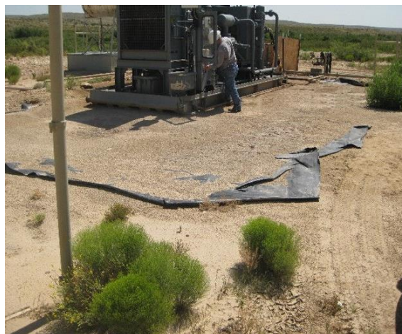
Figure N.5: A layer of sand was placed on this environmental liner to reduce the risk of personnel slipping.
