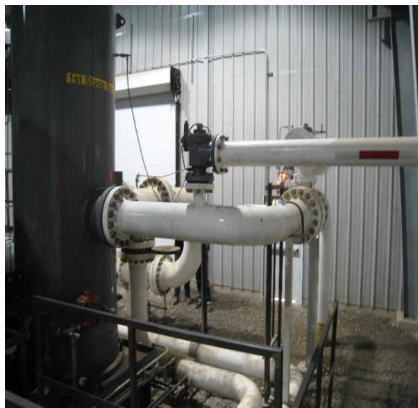
Figure P.6: Pilot-operated PSV located off-skid on suction piping.
