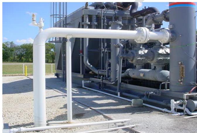
Figure P.2: Example of clear access with minimal trip hazards around a compressor package.
