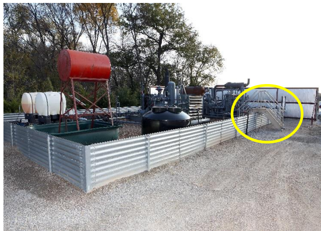
Figure N.4: Although the stairs help personnel scale the environmental wall, service trucks cannot reach the package for maintenance.
