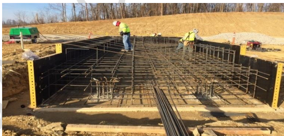
Figure N.14: Typical concrete rebar arrangement with anchor bolt cages.
