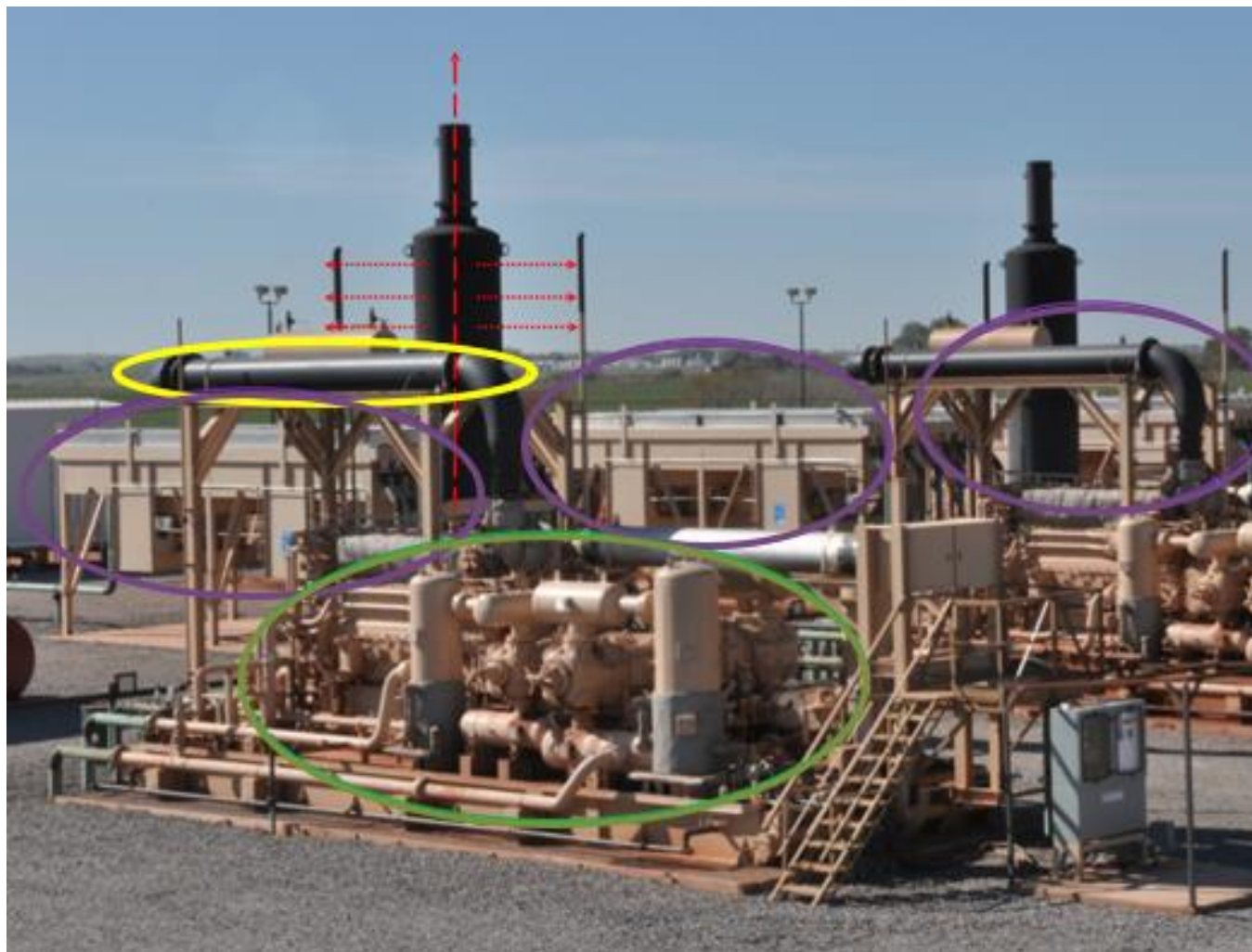
Figure M.1: Examples of the many noise sources in a compressor package - engine exhaust (partly shown in the yellow circle), engine air intake, compressor and cylinders (shown in the green circle), skid piping and pressure vessels (also shown in the green circle), coolers (shown in background within the violet circles), etc.
