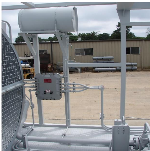
Figure L.6: Example of rigid galvanized steel conduit.
