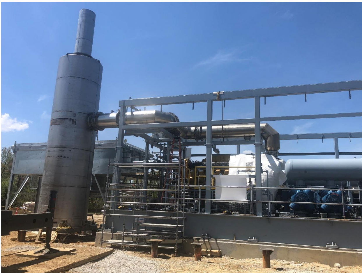
Figure K.2: Example of an insulated exhaust system installed for use inside a skid-mounted building.
