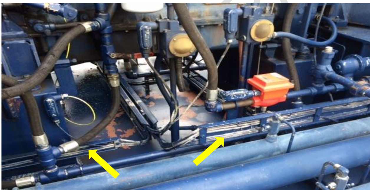
Figure L.8: Armored marine cables routed in cable trays for protection from being stepped on.
