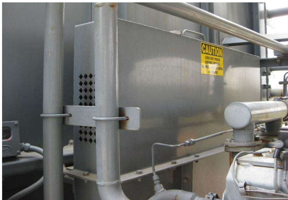
Figure K.1: Example of a well-designed cooler belt-drive guard.
