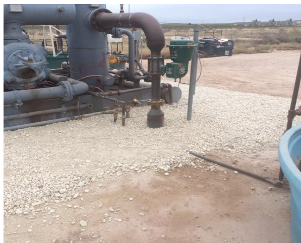
Figure P.3: Example of gravel applied to reduce trip hazard of piping around the package.
