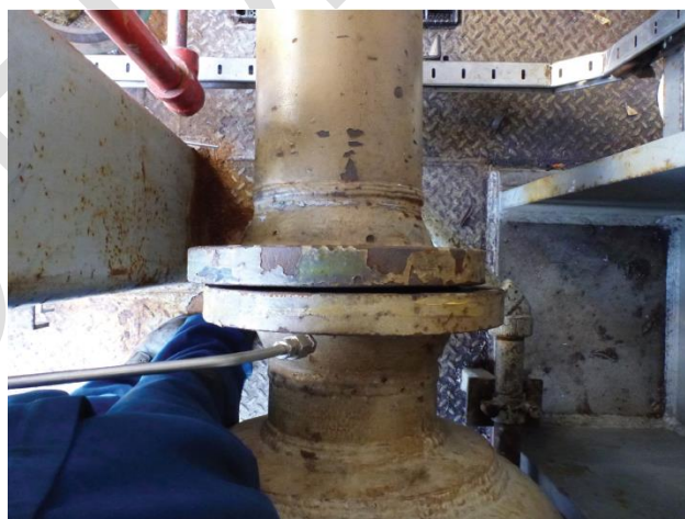
Figure P.13: Assembly of these misaligned flanges will lead to piping strain.
