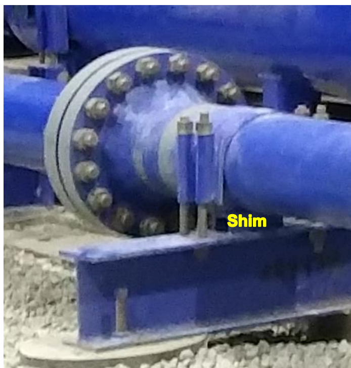
Figure P.15: Example of a shim under a pipe at a clamping location.
