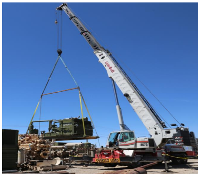
Figure O.2: Complete small compressor package being lifted by a single crane with spreaders.
