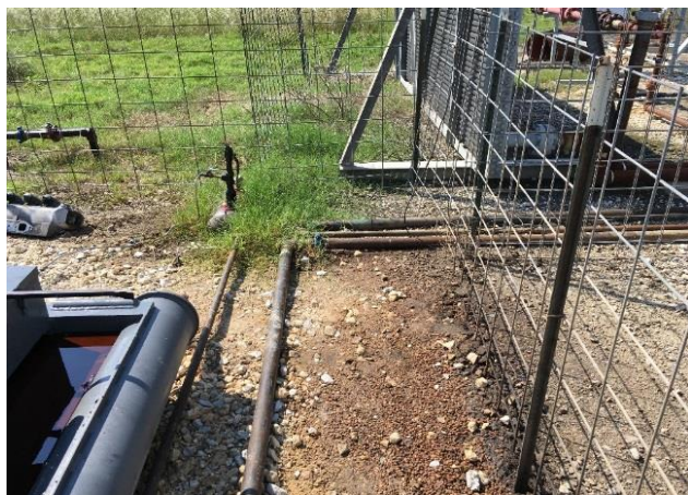
Figure P.1: Example of a trip hazard from piping on the surface around a skid.
