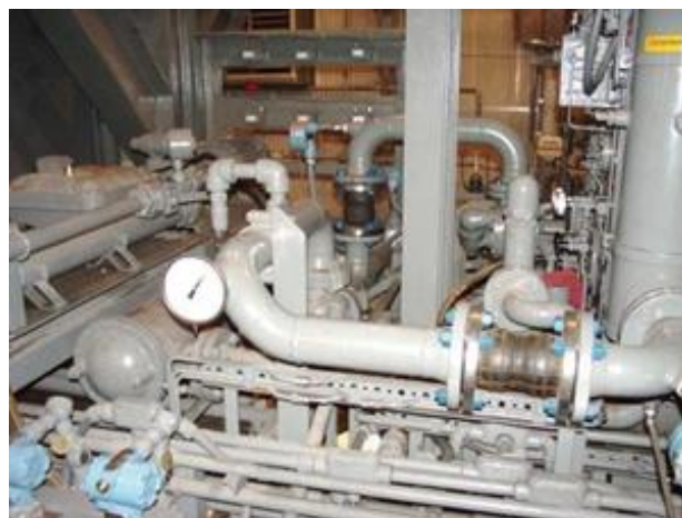
Figure L.2: Another view of the congested packaging that makes maintenance access difficult.
