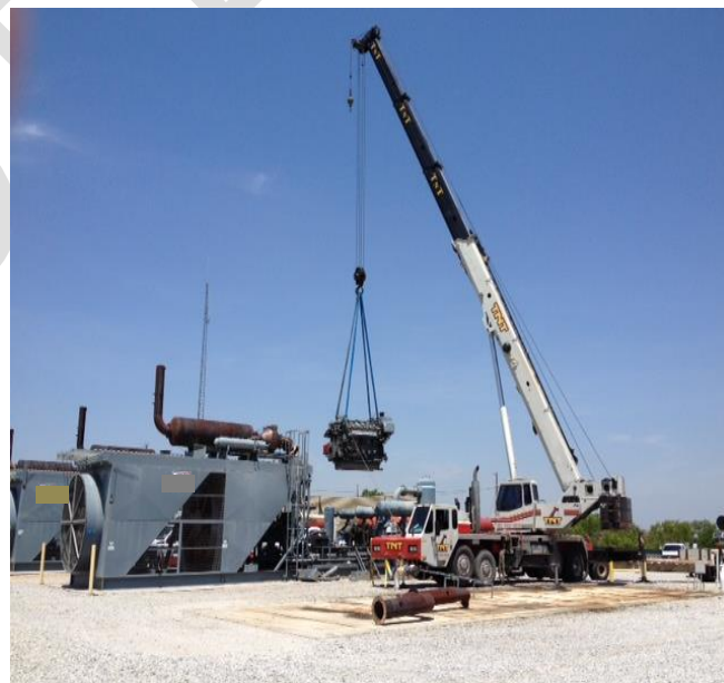
Figure O.5: Separated engine being lifted onto its package already positioned onsite.
