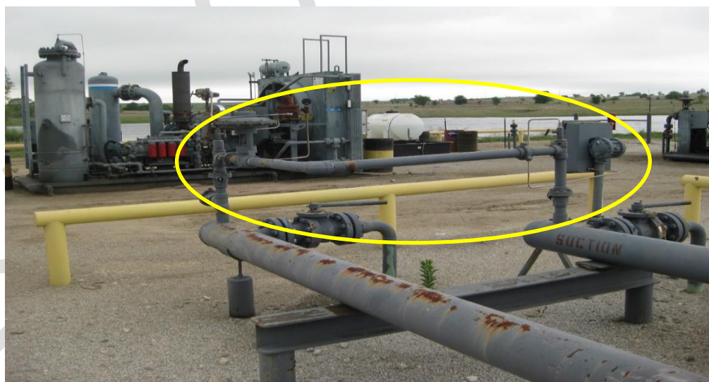
Figure P.10: Recycle system connecting suction and discharge headers at a field gas compressor station.
