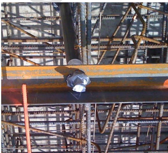
Figure N.17: Long sleeve around the anchor rod up to the top of concrete, with protection to keep concrete out of the sleeve and away from threads during concrete placement.
