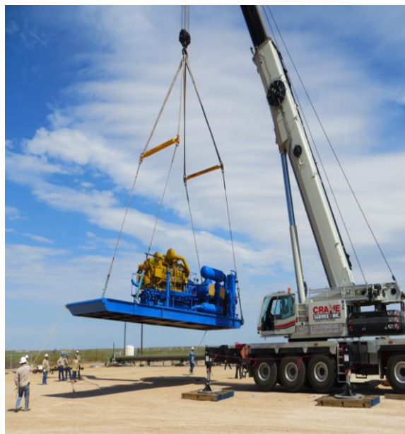
Figure O.4: Package being lifted at site with cooler removed.
