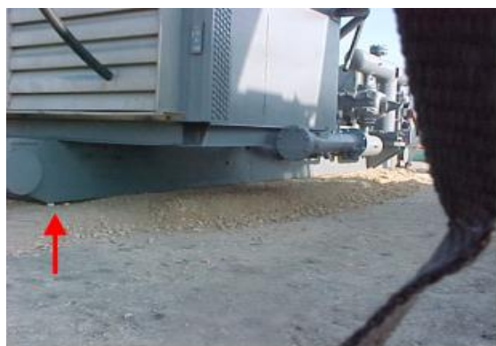
Figure N.25: End of skid not supported.
