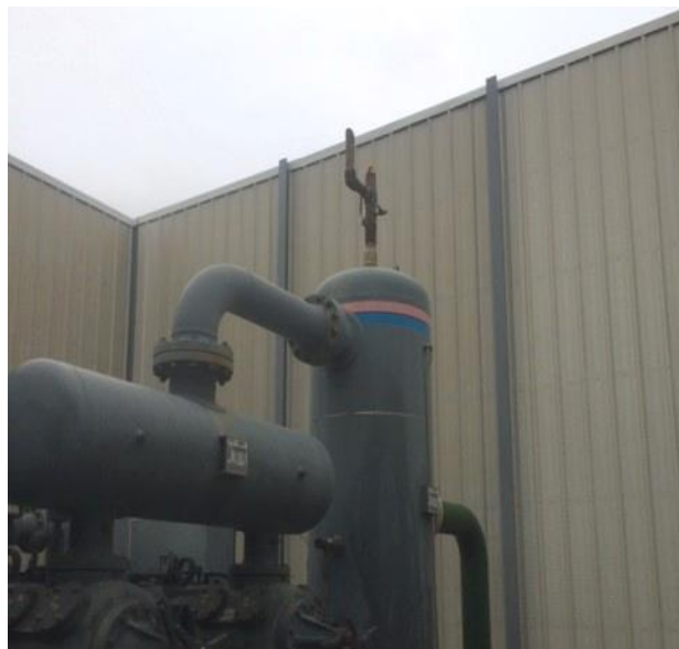
Figure P.5: PSV mounted on top of suction scrubber with short vent line to atmosphere.
