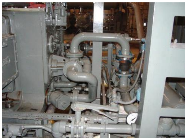
Figure L.1: Example of a package with excessive congestion that inhibits access for maintenance.
