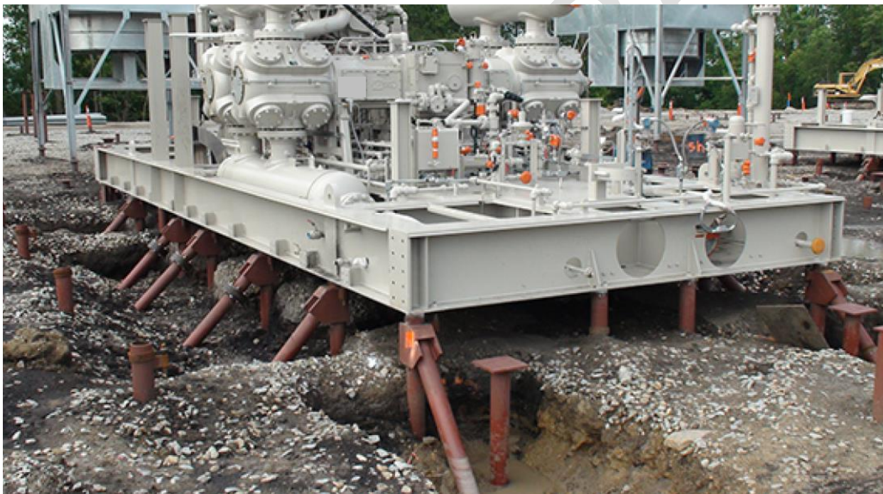
Figure N.20: Screw pile mounted compressor package.
