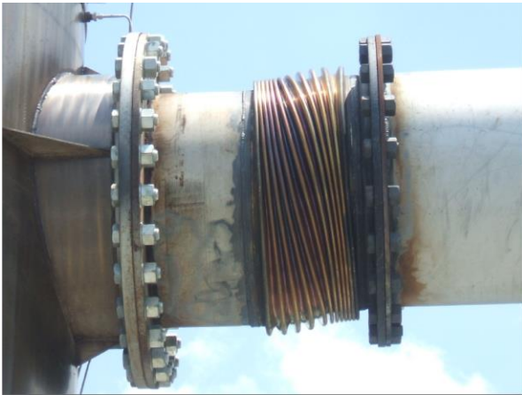
P.19: Horizontal flexible exhaust line element with excessive misalignment and loading.
