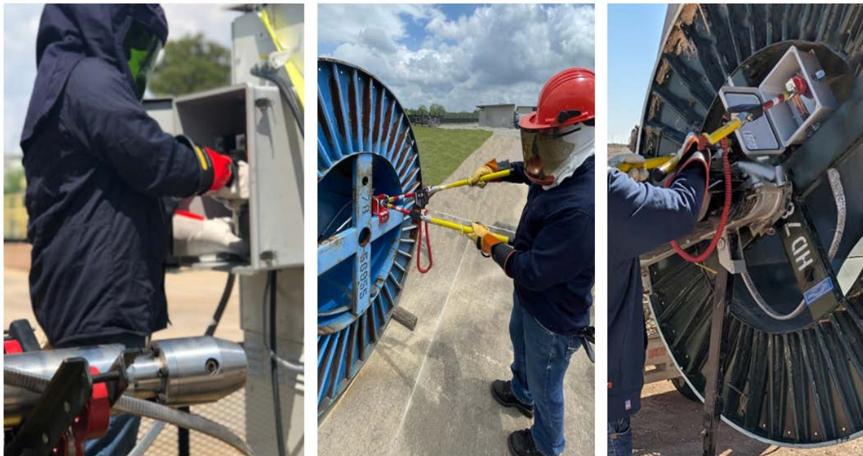
Figure K.6—PPE usage and volt stick at shunt.
