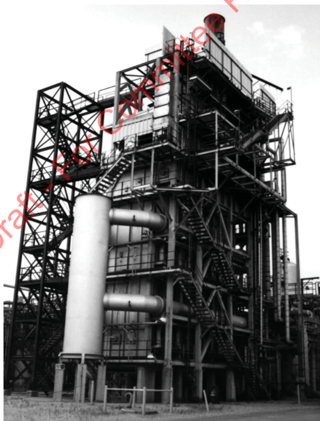
Figure 3—One Type of Steam-Methane Reforming Furnace
