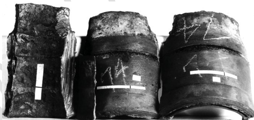
Figure 25—Fitting and Tube that Have Leaked in the Roll
