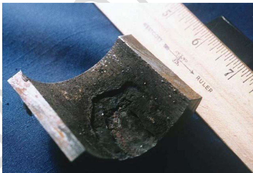
Figure 14—Localized Tubing Wall Loss Caused by Caustic Gouging
