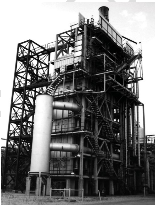
Figure 3—One Type of Steam-Methane Reforming Furnace
