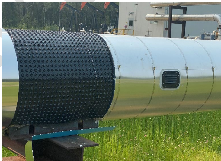
Figure 41 - Perforated and dimpled Insulation drying wrap system
