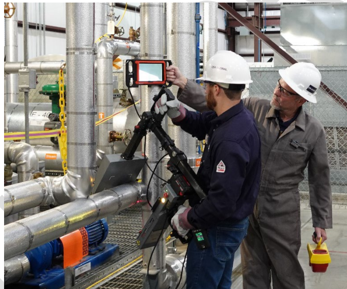
c) RTR Operators performing a CUI pipe examination
