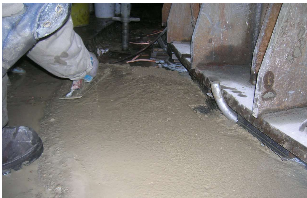
Figure 63—Final Grout Stage
