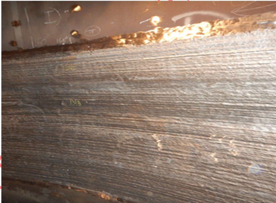
Figure 68—Finished Structural Overlay Deposit
