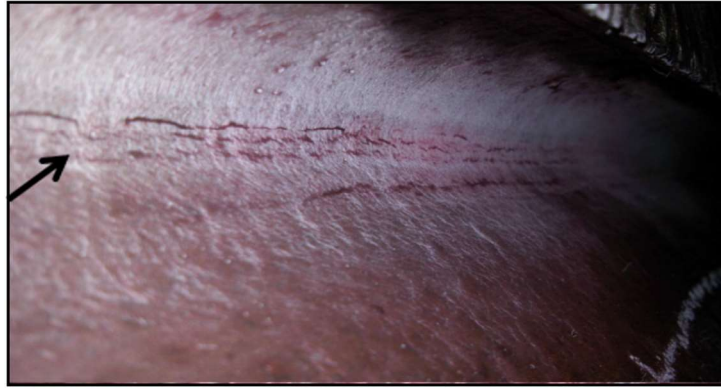
Figure 12—PT from the Outside Surface Highlighted Cracks in the Vicinity of the Skirt Attachment Weld
