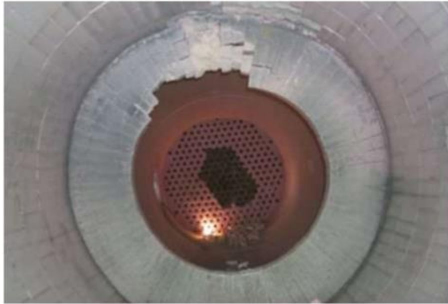
Figure B.8– Pinch Spalling of Brick in SRU Reaction Furnace.
