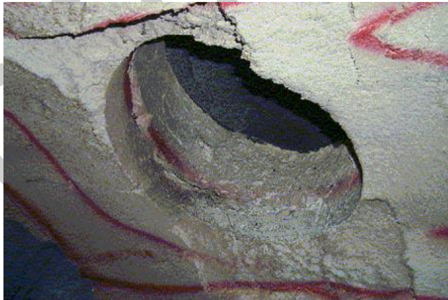
Figure B.11 – Severe Cracking of Castable Refractory Around a CO Boiler Nozzle
