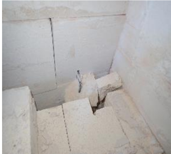
View of failed tie back
