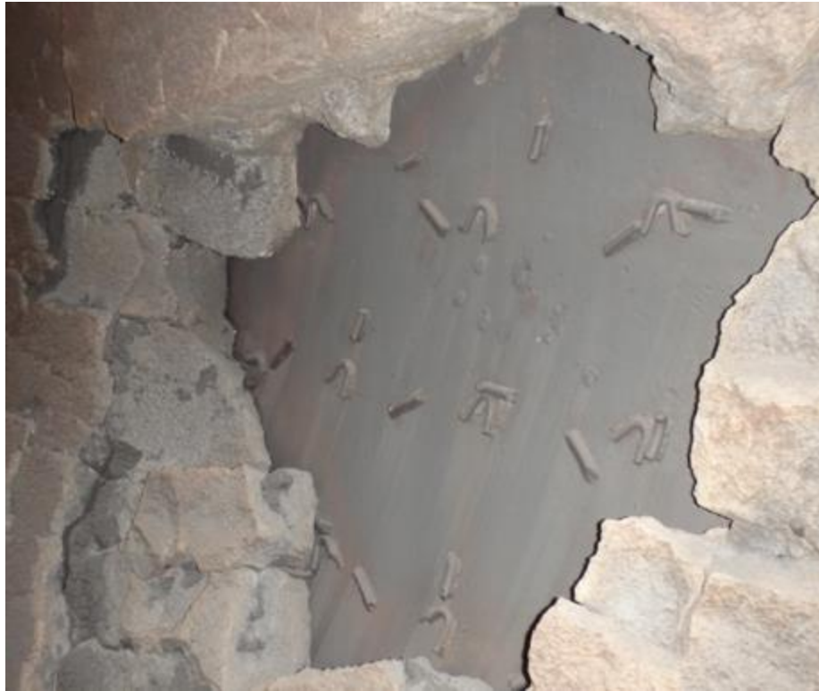
Figure B.21 – Failure of Anchor Legs Above Attachment Weld
