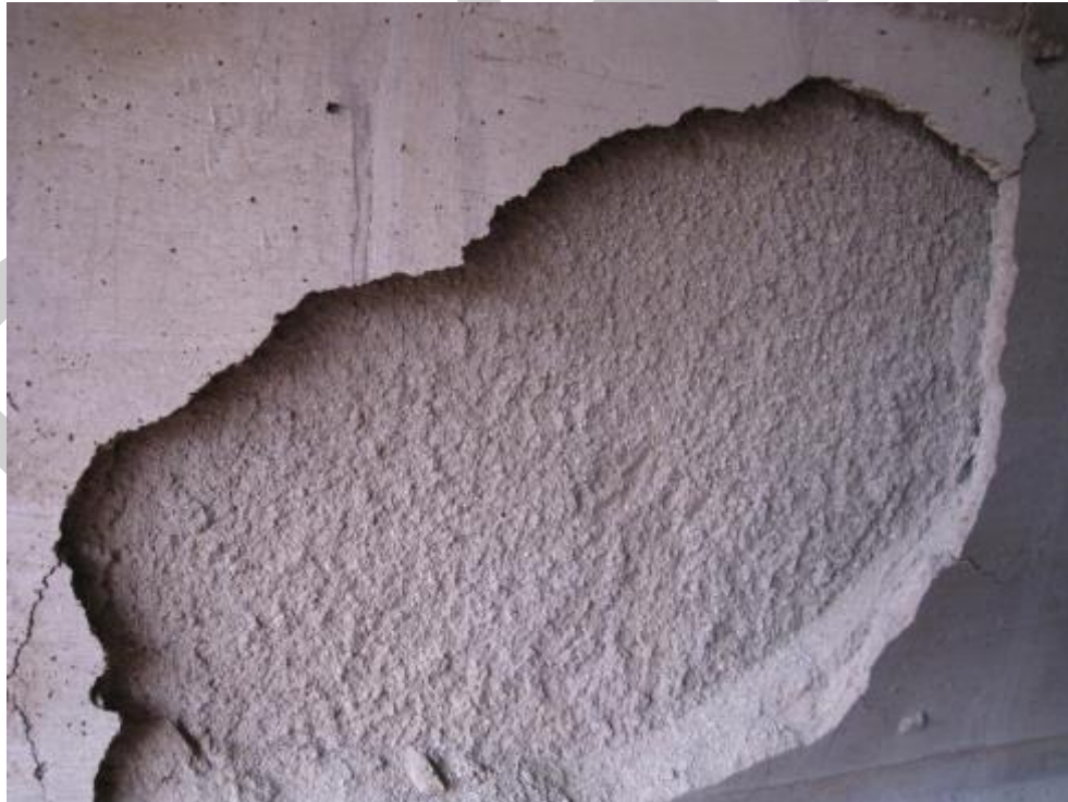
Figure B.16 – Alkali Hydrolysis
