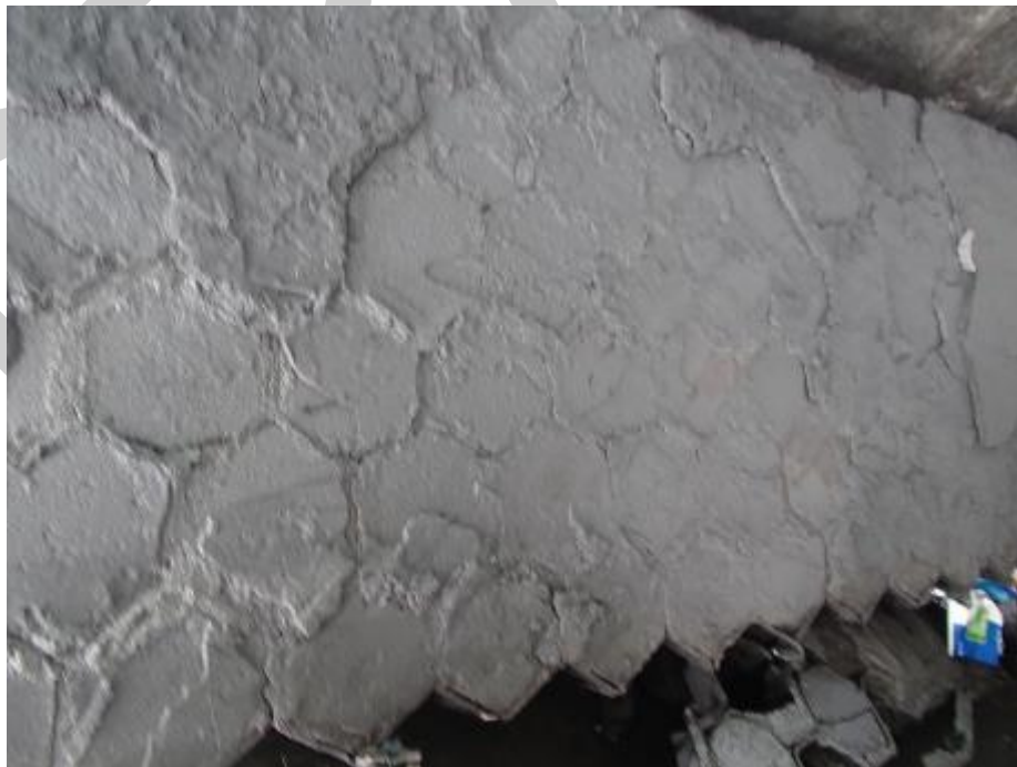
Figure B.22– Sheets of Hex Falling Away Due to Insufficient Welding.
