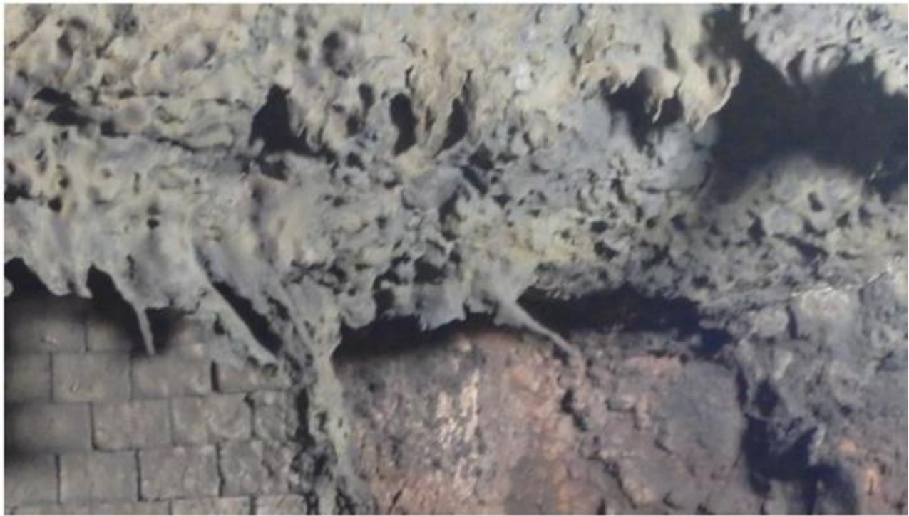
Figure B.15– Slag Attack
