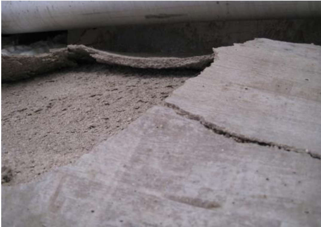
Figure B.17 – Alkali Hydrolysis
