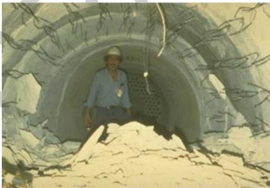
Figure B.5 – Explosive Spalling
