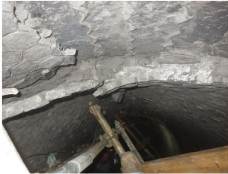
Figure B.6– Spalling of Hexmesh Caused by Coke Jacking
