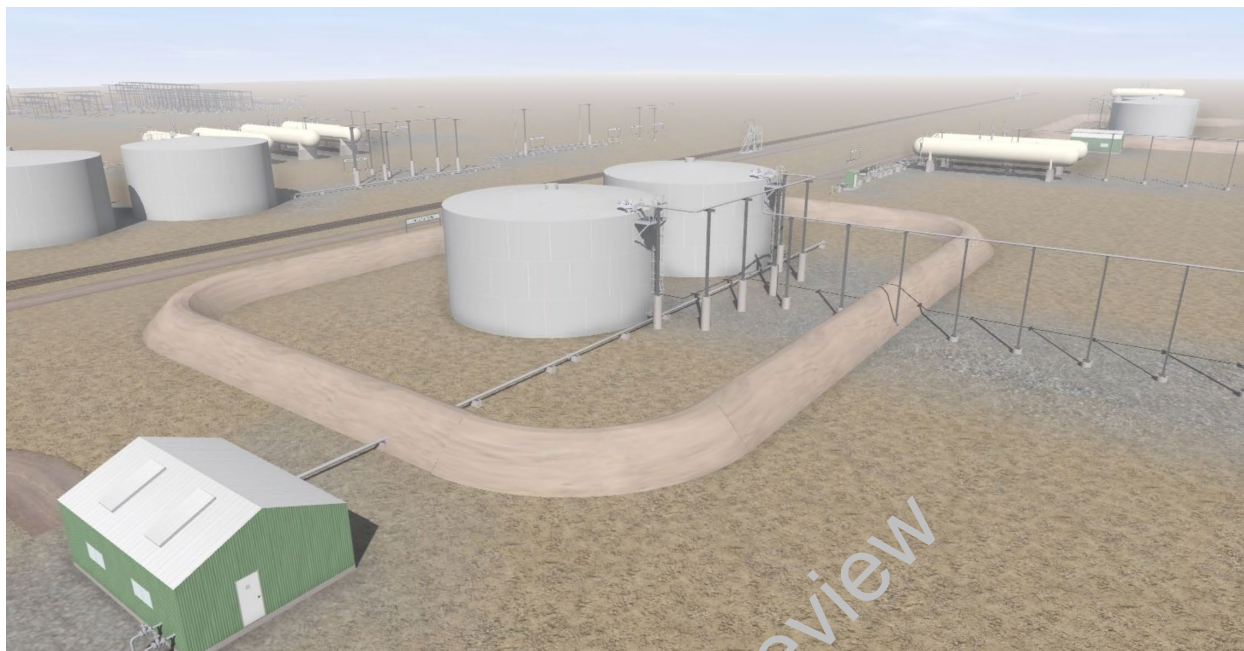
Figure 1 Secondary Containment Berm
