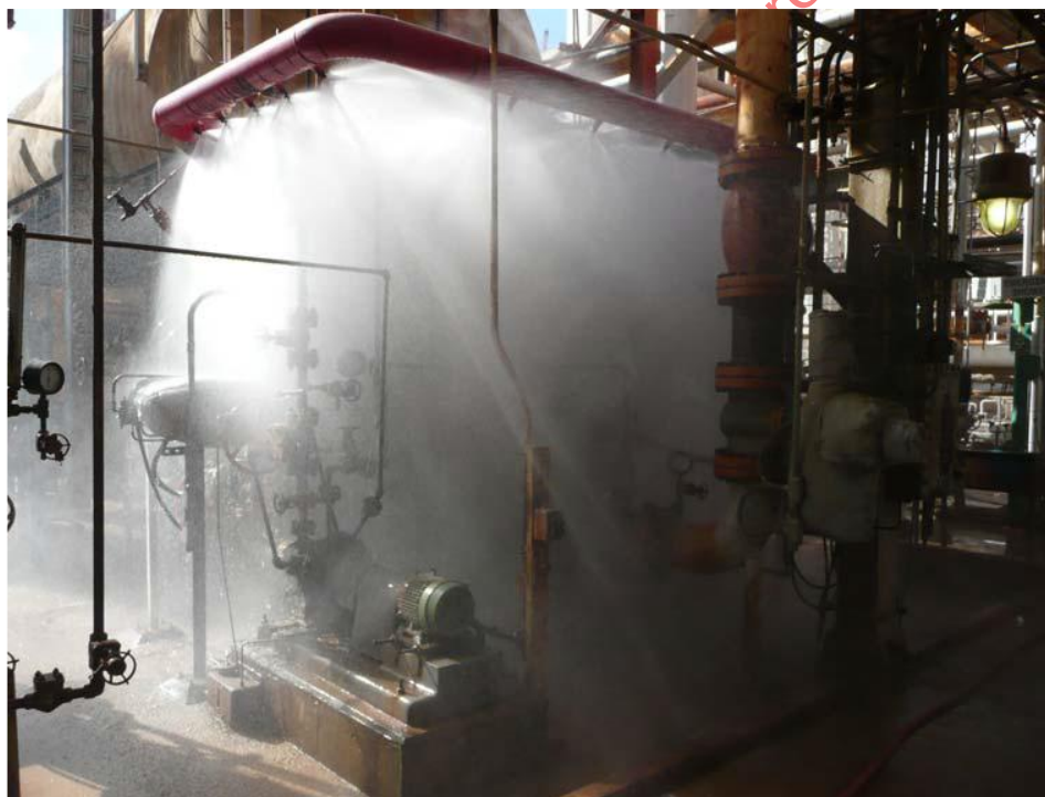
Figure K.5—Example Equipment Deluge System
