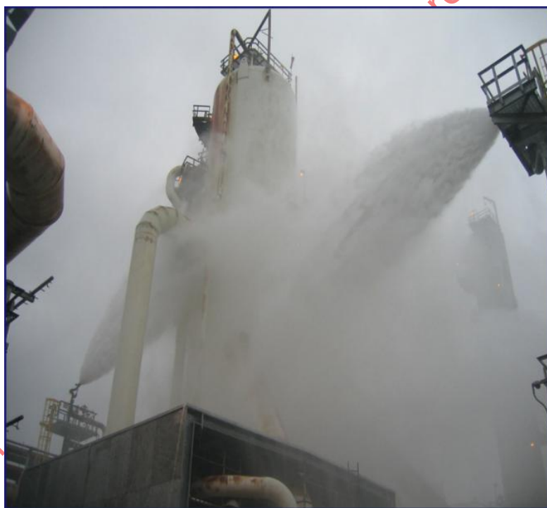
Figure K.4—Example Aim-and-Shoot Water Mitigation System
