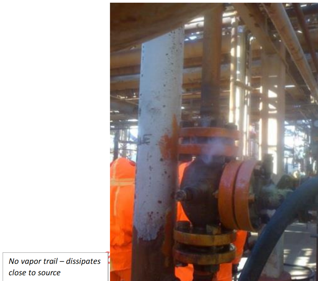
Figure E.3— Example of Category 3 Leak
