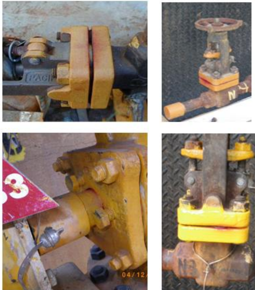
Figure E.1—Examples of Category 1 Leaks
