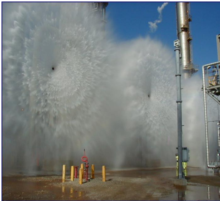
Figure K.3—Example Water Wall
