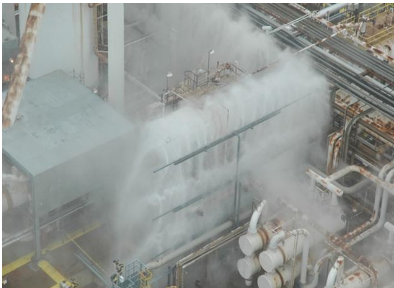
Figure K.2—Example Water Curtain
