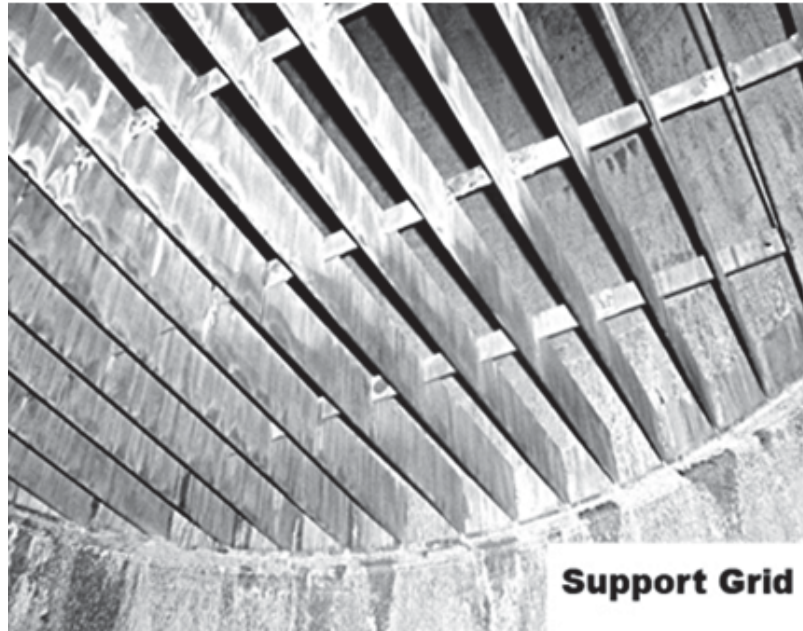
Figure B.46 - Support Grid from Below
