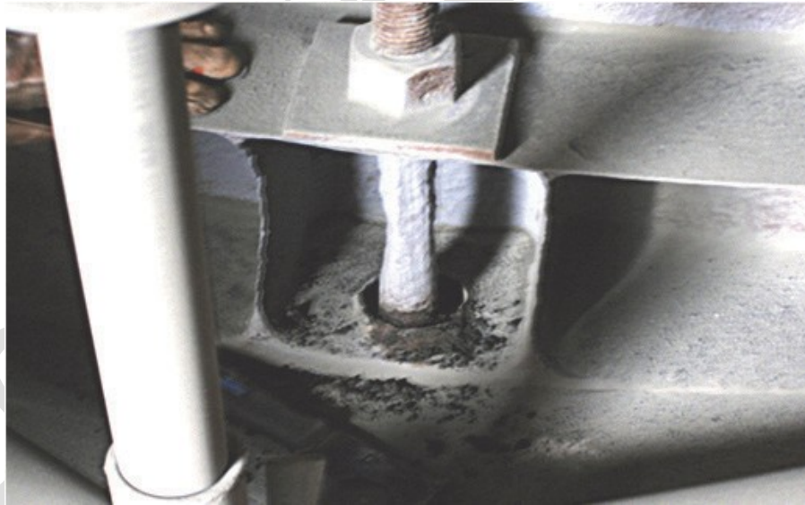
Figure B.18 - Corroded Anchor Bolting
