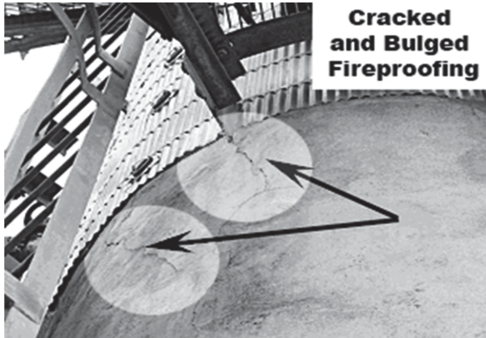
Figure B.19 - Cracked and Bulged Fireproofing
