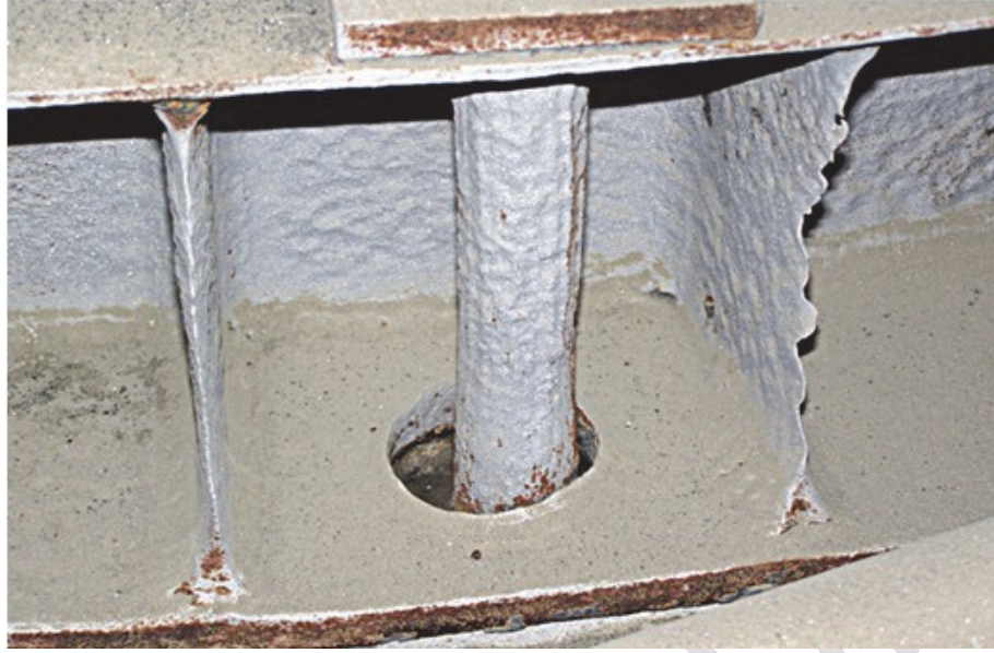
Figure B.17 - Corroded Anchor Bolting
