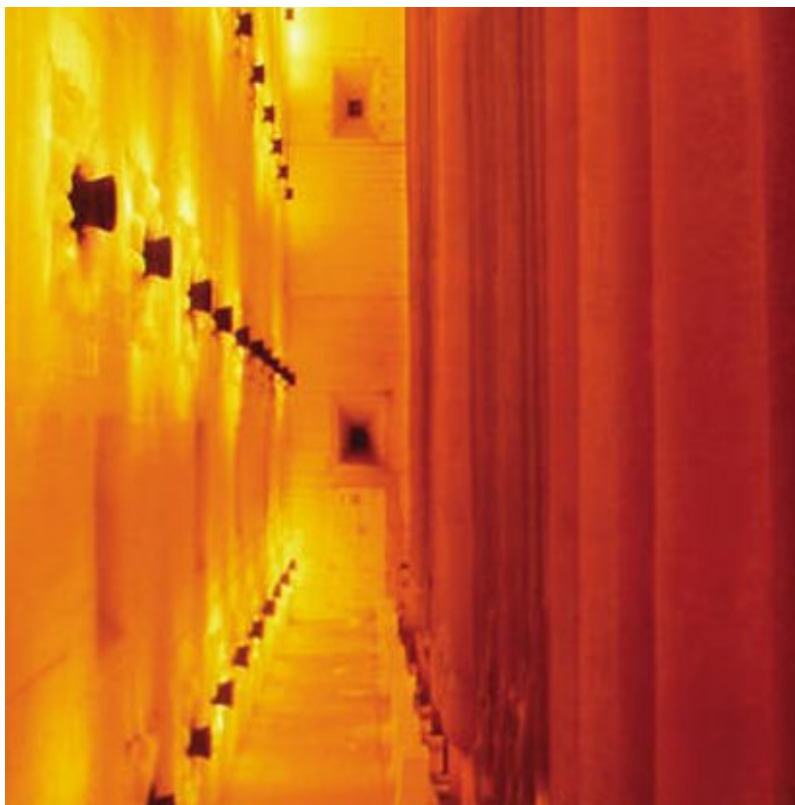
Figure D.1—Side Wall Fired Reformer Furnace in Operation
